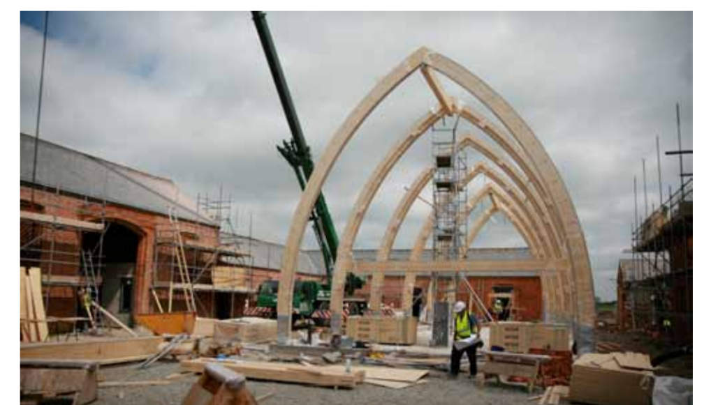
View of Mucknell Farm during construction
