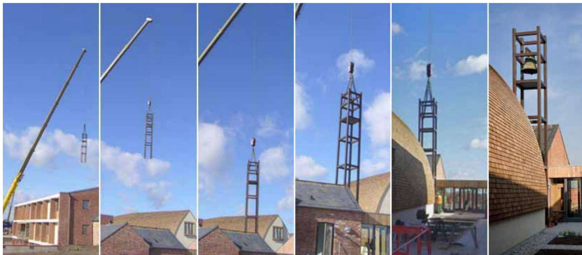
Installation of the bell tower: during the works Below: external view of the Oratory within the courtyard
